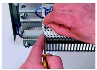
Connecting a lead to the spring-loaded terminals
